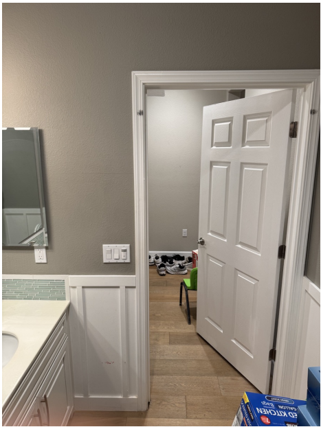
P05 / Bathroom doorway / outward swing
