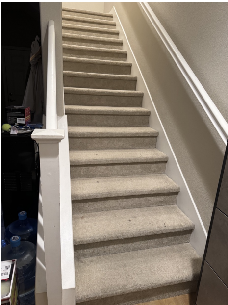
P06 / Stair railing becomes solid wall
